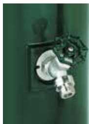
-32 compression type, hose end and VB
